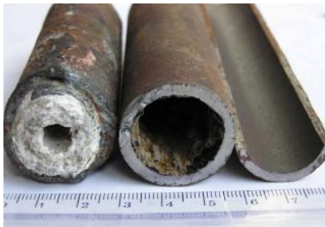
Fig. 2. Coil of steam generator with the layer of fur
